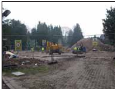
The building site previously occupied by Harestone House.
